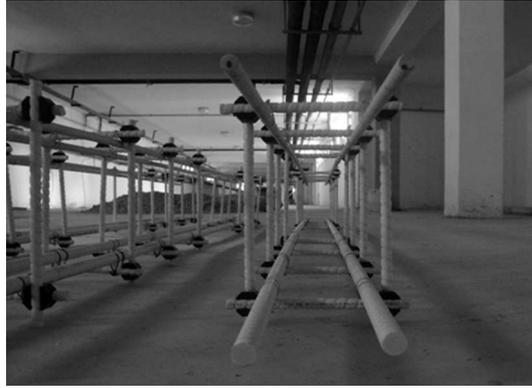
Fig. 1. GFRP bars reinforcement and the beam cross section
